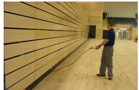
Type V - Traveling unit which allows movement as a complete bank, forwards and backwards, from its stored position.
