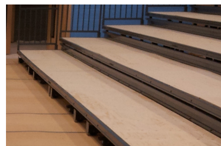
3/4" plywood deckboards (for finishes, see page 4).
