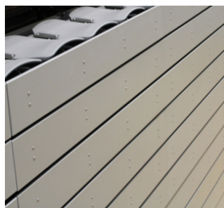
Fascias with plain melamine finish. (Those shown are through bolted for additional strength in a ball sport venue.)
